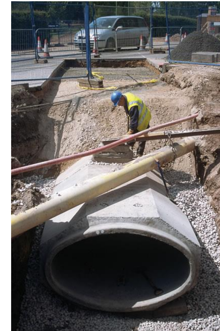
Typical example of a new culvert
