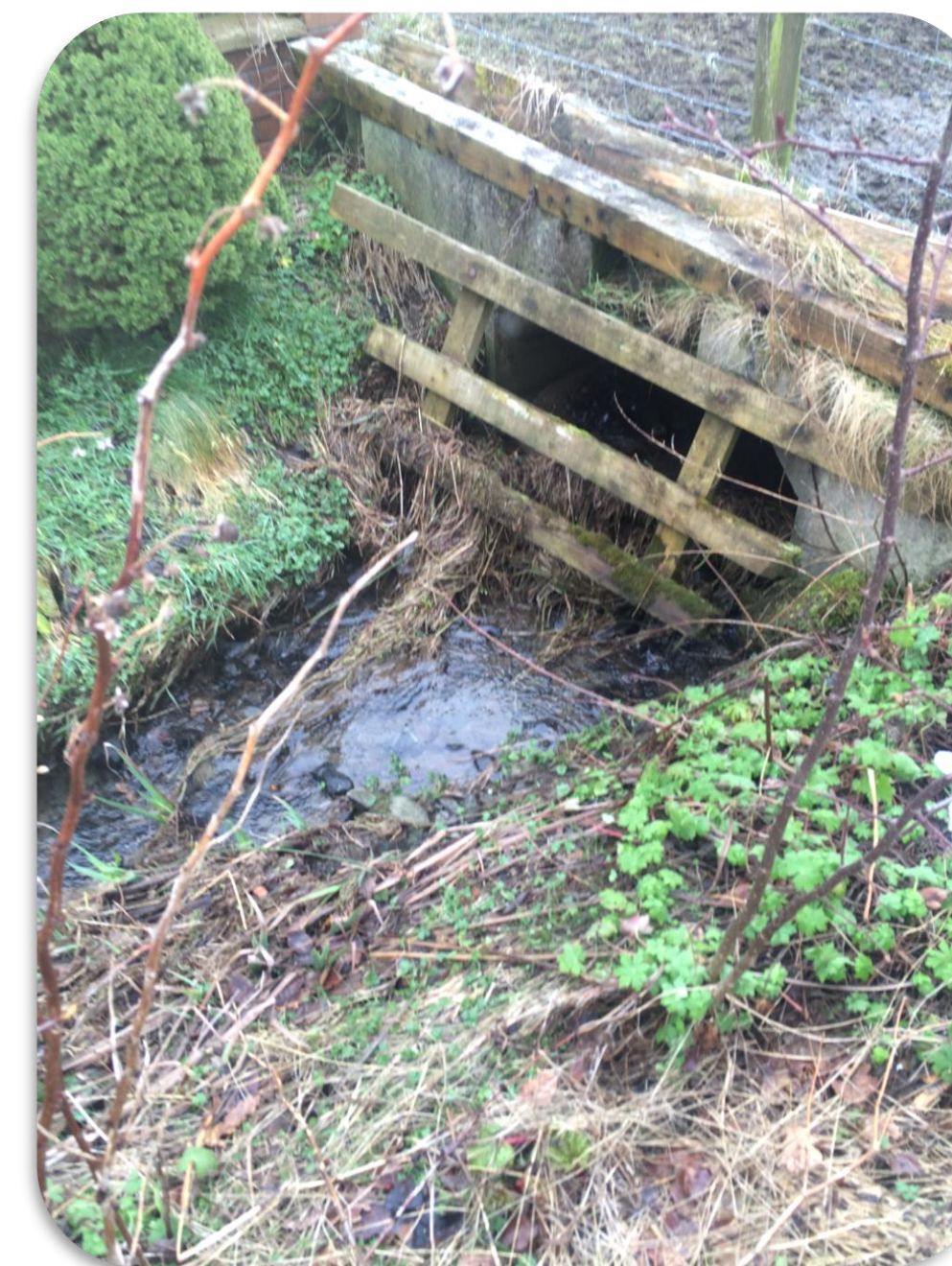
Bridge on diversion channel
