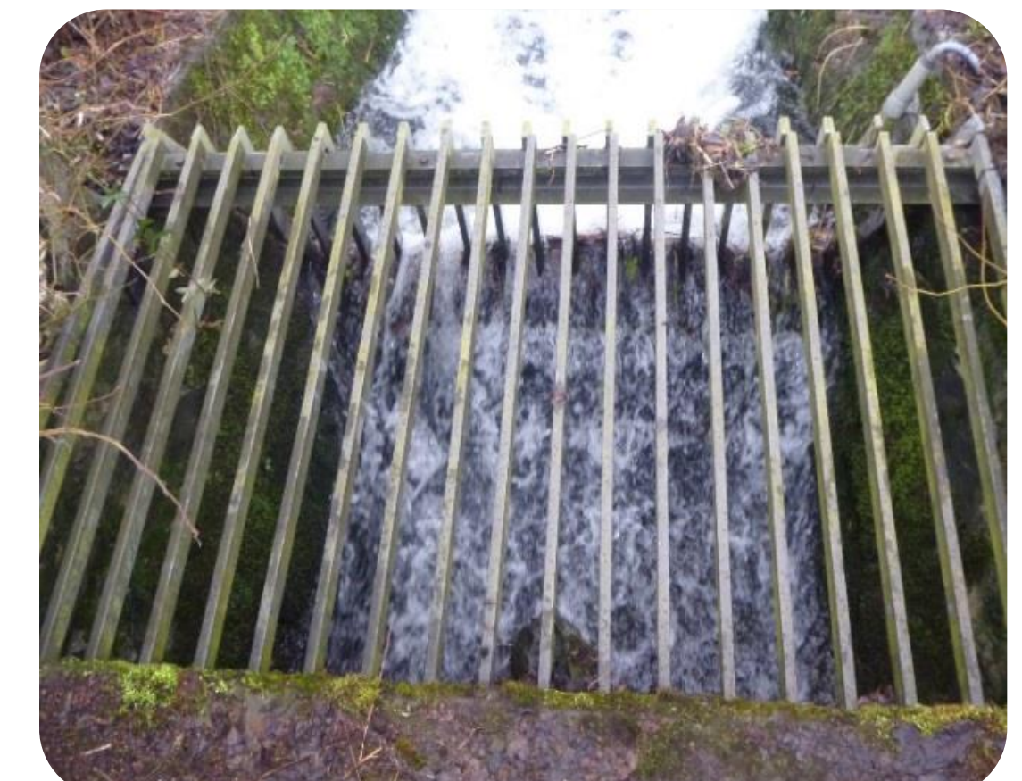
Screen on Edderston Burn culvert
