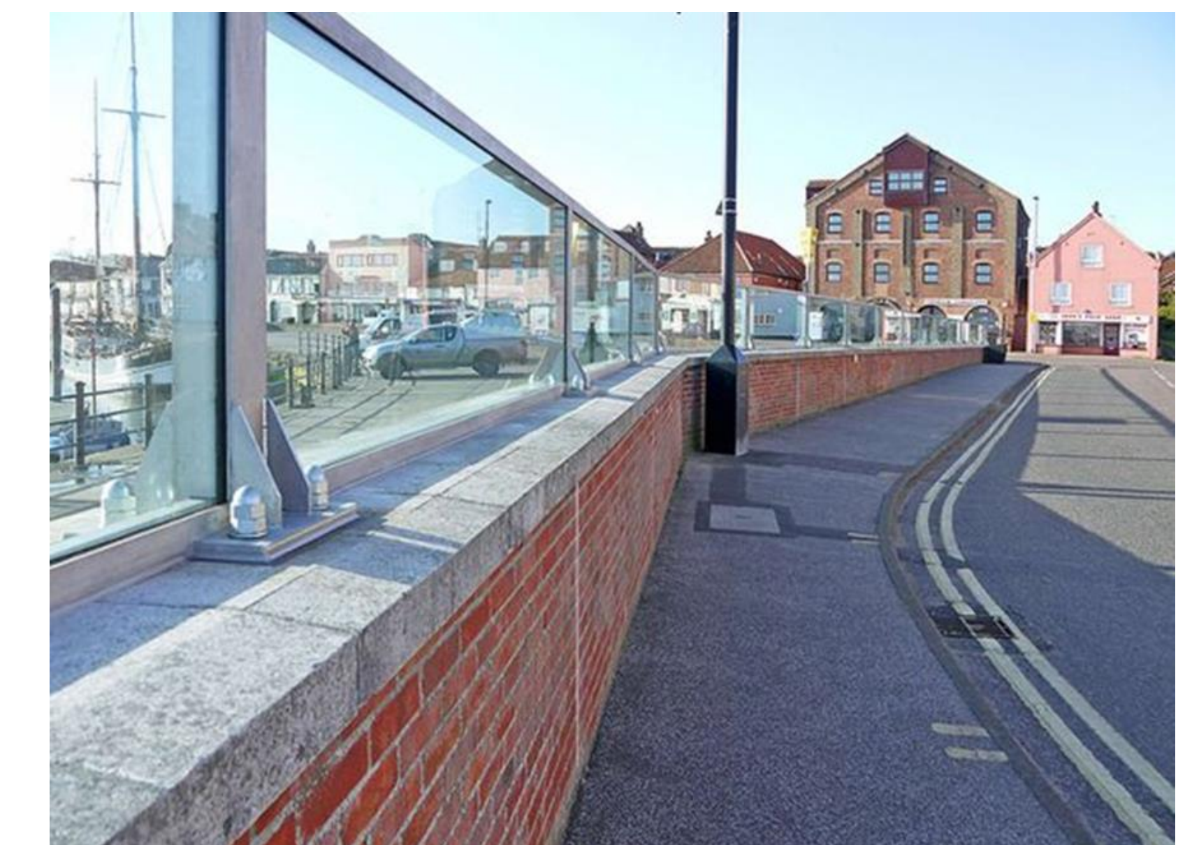
Typical example of a flood wall
