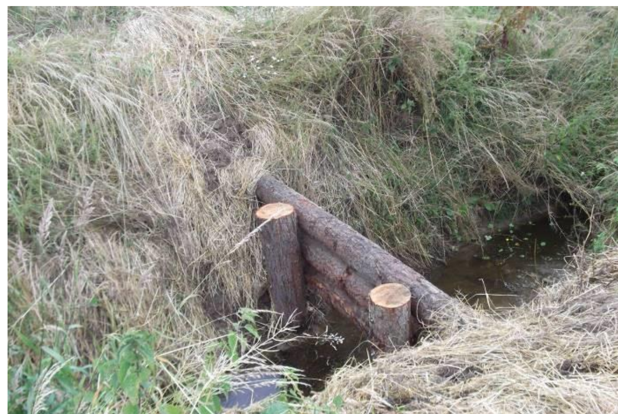
Typical example of in-channel debris barrier
