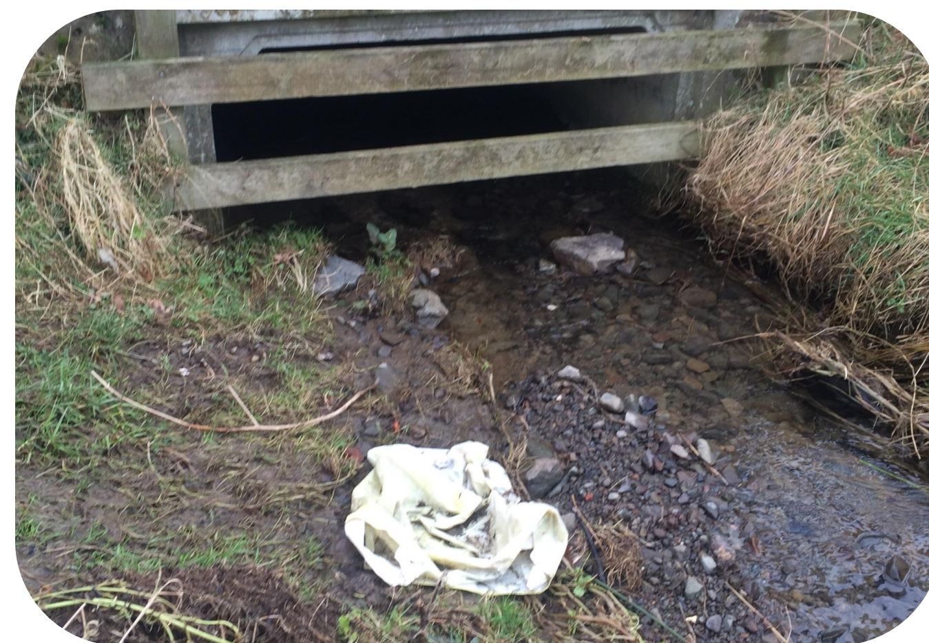
Bridge on diversion channel
