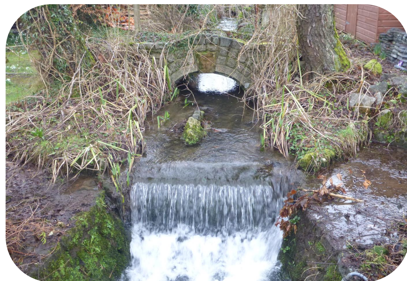
Bridge and weir on approach to Edderston Burn Culvert
