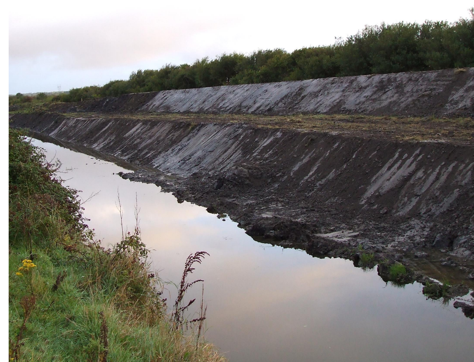
Typical example of channel widening
