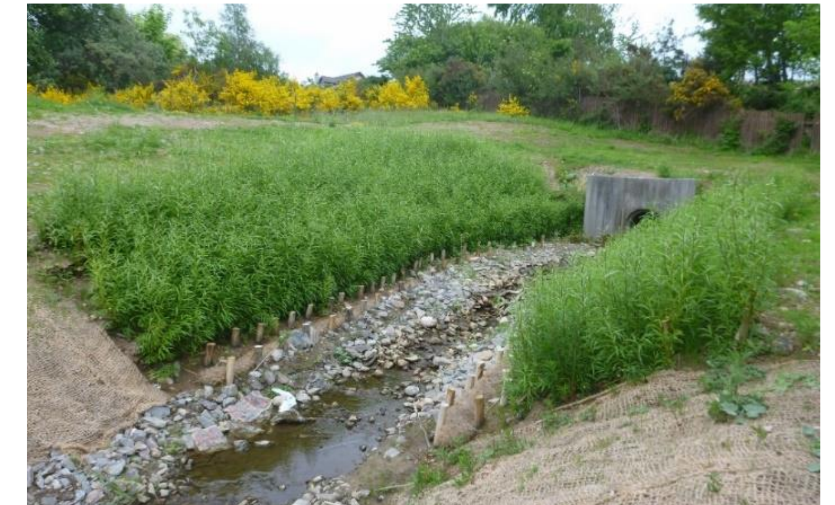
Typical example of channel deepening
