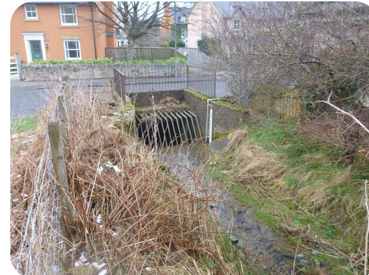
Diversion channel wingwall tie-in
