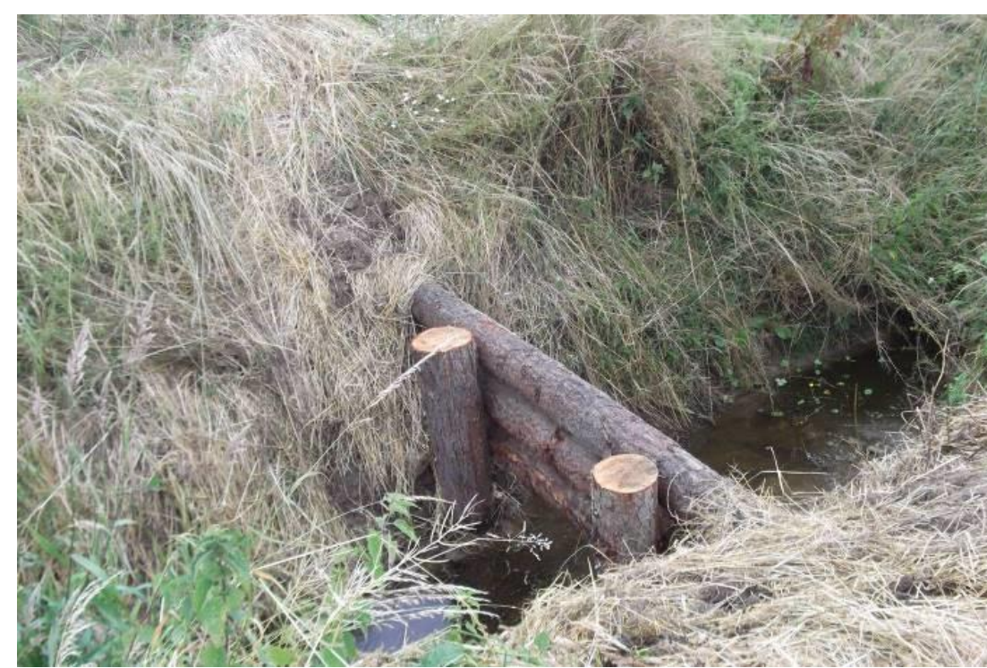
Typical example of in-channel debris barrier
