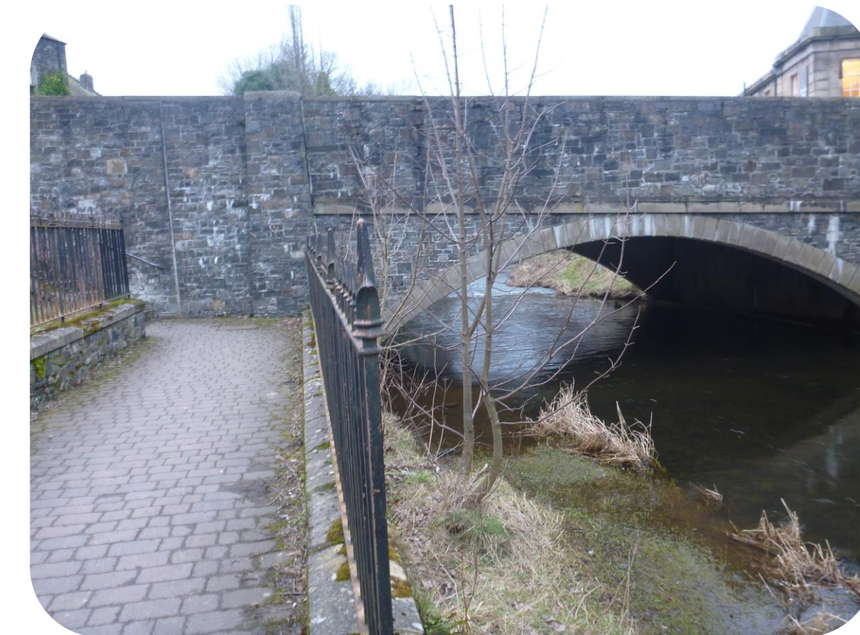
Bridges capable of constraining flood flows
