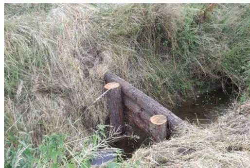
Typical example of in-channel debris barrier
