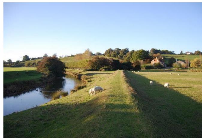
Typical example of a flood embankment
