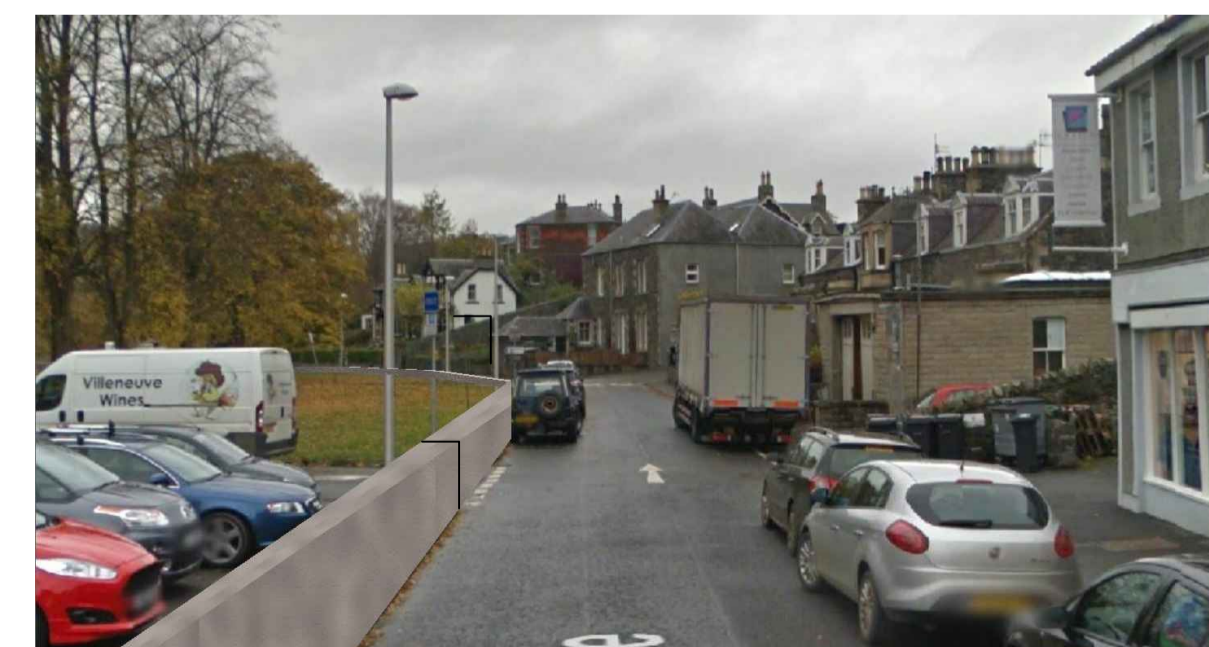
SECTION B-B Artist interpretation of wall with indicated gate for car park
